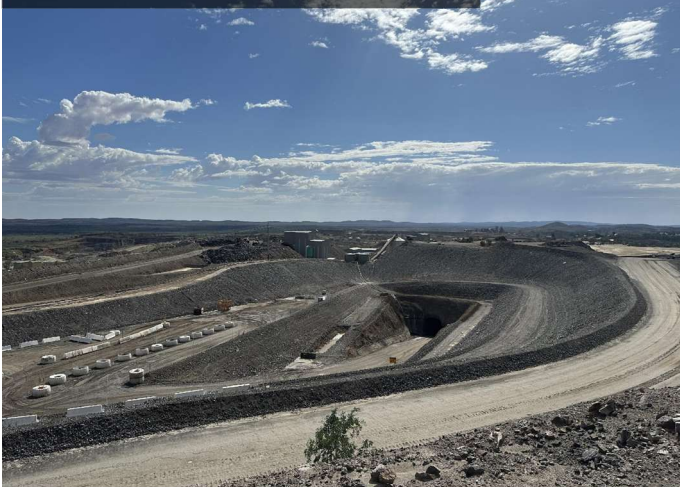
New portal & decline (2022)
