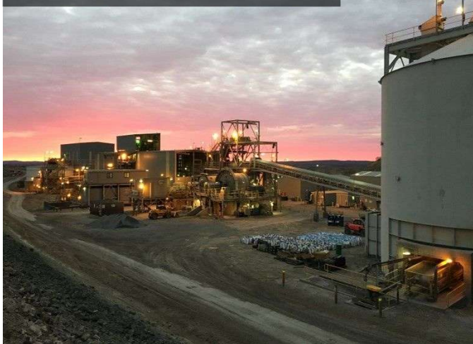
750,000tpa capacity processing facility
