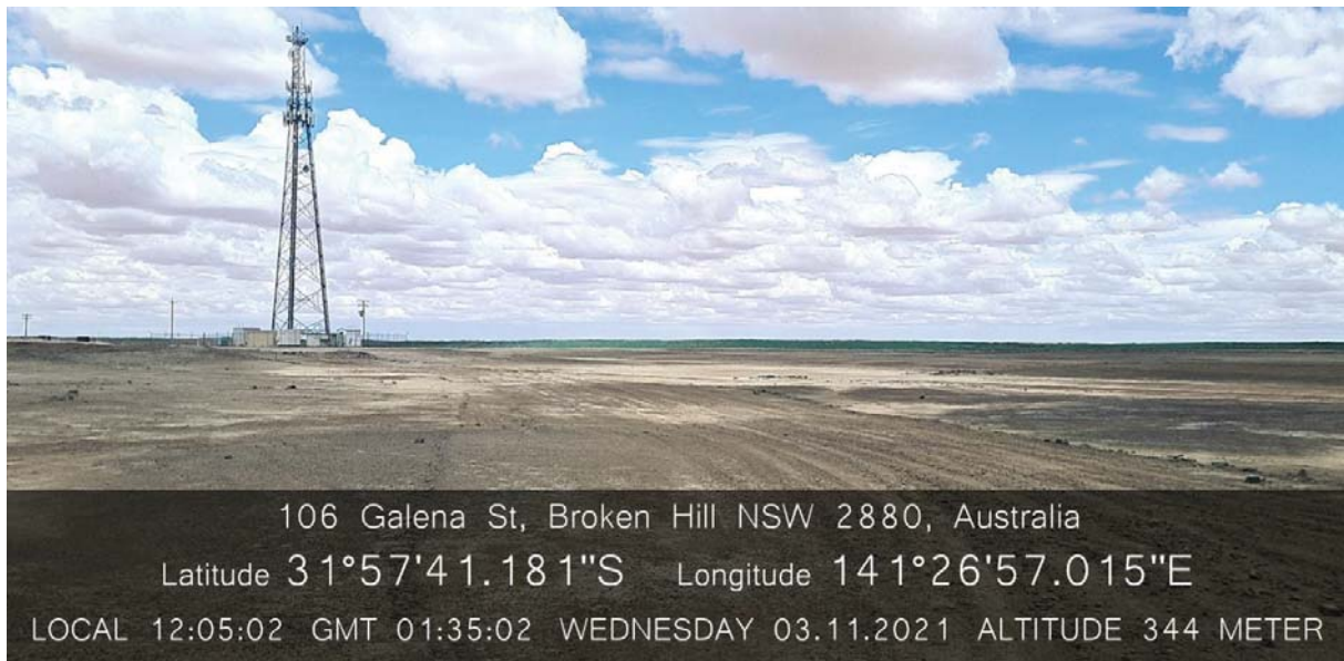
Photograph 1.1 Vodaphone communications tower
